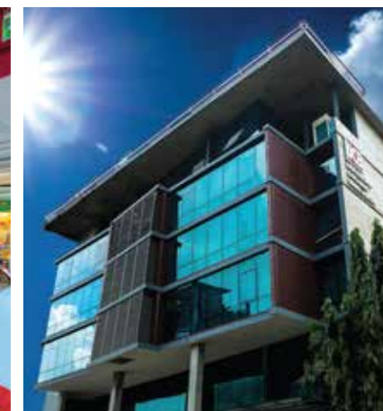
LOCATION SA Tower, 1 Gulshan Avenue, Dhaka
